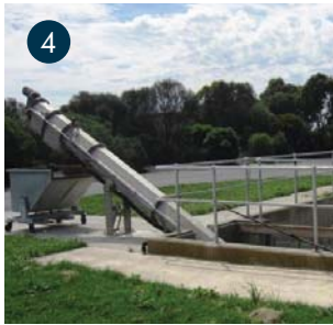
3. TYPICAL SET UP FOR A SPIROGUARD® CS SCREEN
