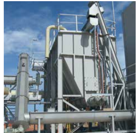
72° and 40° inclined OK trough sludge conveyors
