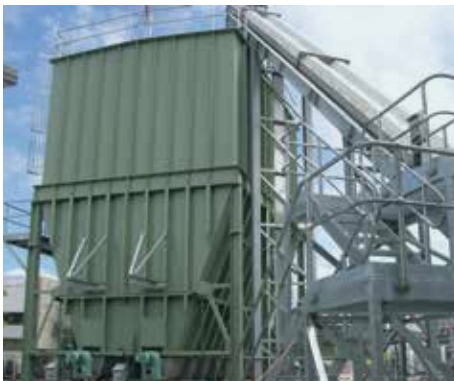
Live-bottom Silo installation
