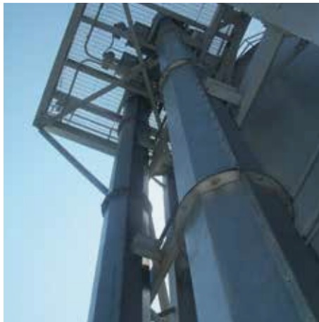
Typical two stage vertical lift sludge conveyors feeding a storage silo
