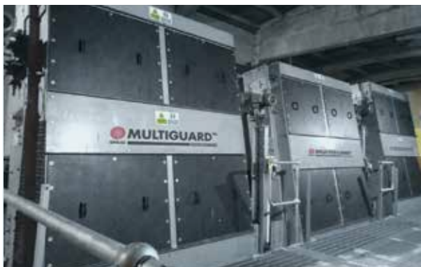
MULTIGUARD™ screens installation
