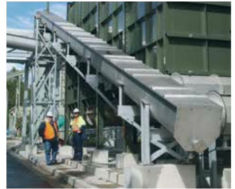
High capacity sludge outloading system
