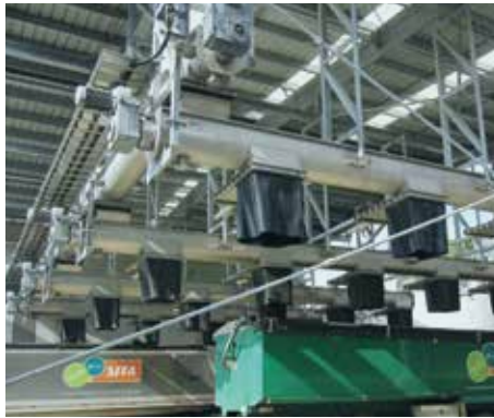
Truck outloading system
