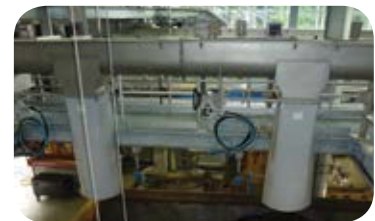
Truck outloading system
