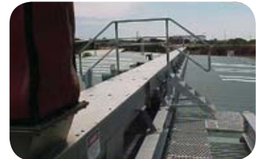
Long continuous sludge run
