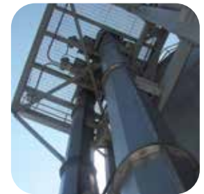
Typical two stage vertical lift sludge conveyors feeding a storage silo
