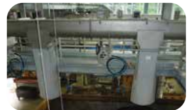
Truck outloading system
