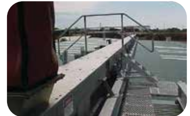
Long continuous sludge run
