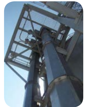
Typical two stage vertical lift sludge conveyors feeding a storage silo
