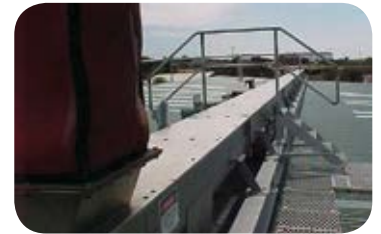
Long continuous sludge run
