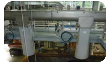
Truck unloading system
