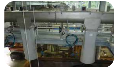
Truck unloading system
