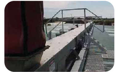
Long continuous sludge run
