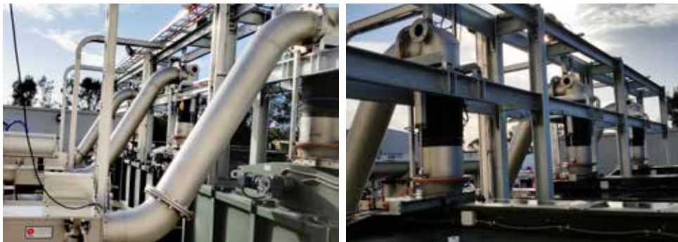
SPIROWASH® and SPIROTAINER®: Screenings washing and storing
