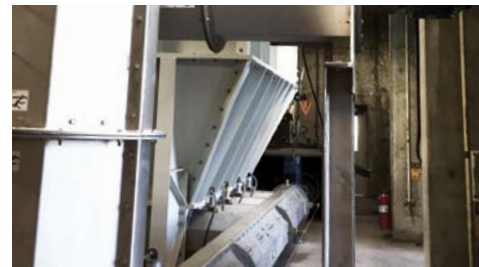
Live-Bottom Silo & Cross Collector
