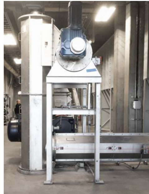
Horizontal & Vertical Sludge Conveyors
