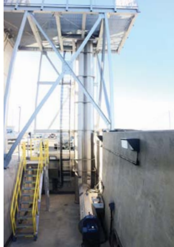
Cross Collector & vert. conveyor
