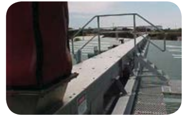
Long continuous sludge run
